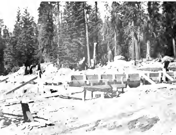
Bunkhouse foundation forms in place, Sept. 18
